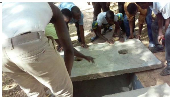
Installation de latrines
